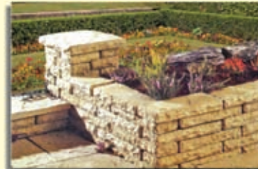
Rock Faced Dry Walling
